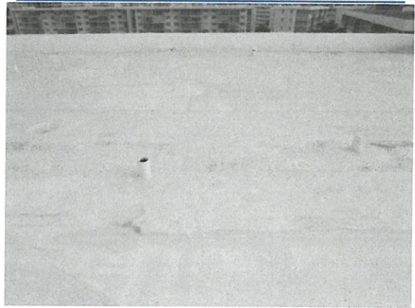
Reinforced Concrete Roof Deck
