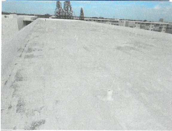
Reinforced Concrete Roof Deck
