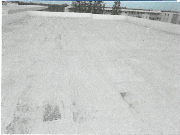
Reinforced Concrete Roof Deck
