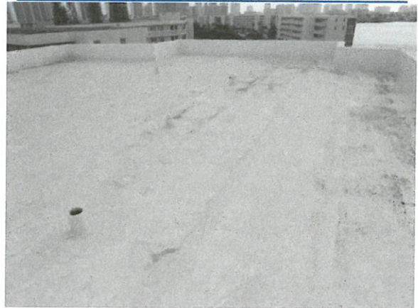
Reinforced Concrete Roof Deck
