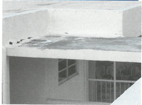
Reinforced Concrete Roof Deck
