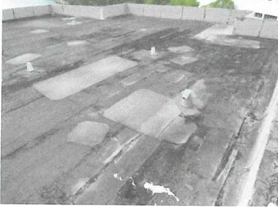
Reinforced Concrete Roof Deck
