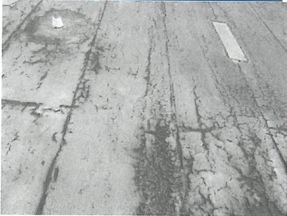
Reinforced Concrete Roof Deck
