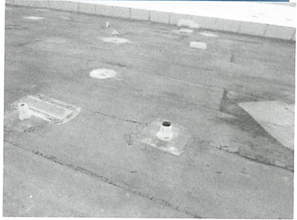
Reinforced Concrete Roof Deck
