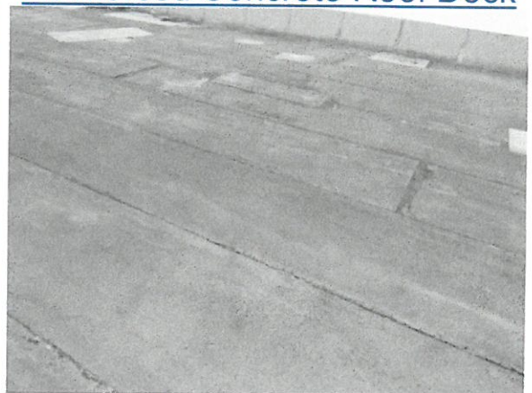
Reinforced Concrete Roof Deck
