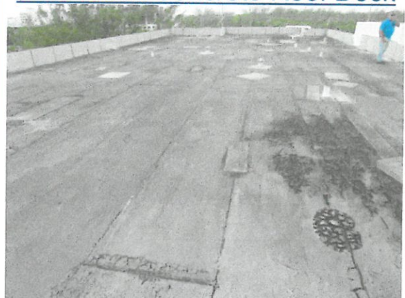
Reinforced Concrete Roof Deck
