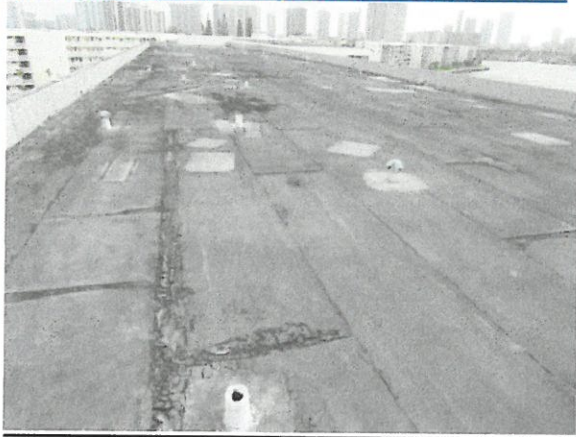
Reinforced Concrete Roof Deck
