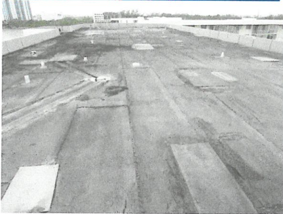
Reinforced Concrete Roof Deck
