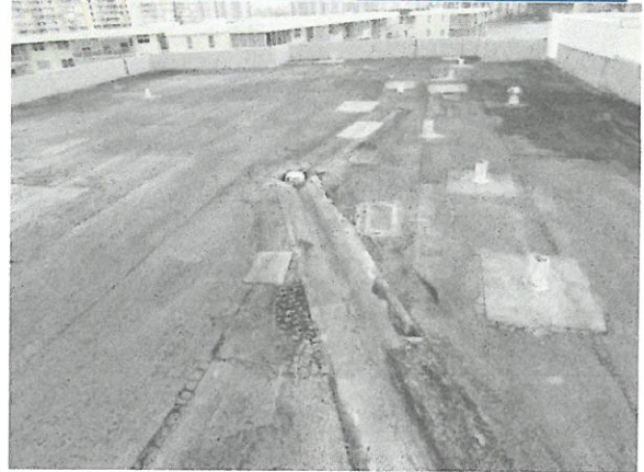
Reinforced Concrete Roof Deck
