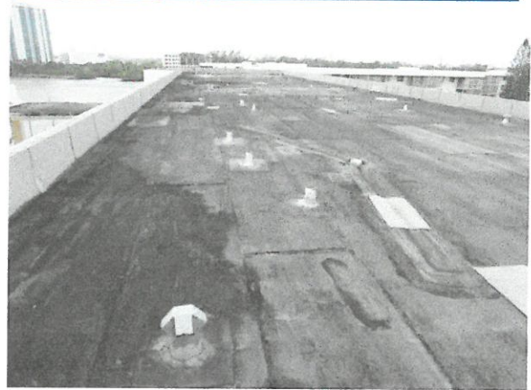
Reinforced Concrete Roof Deck
