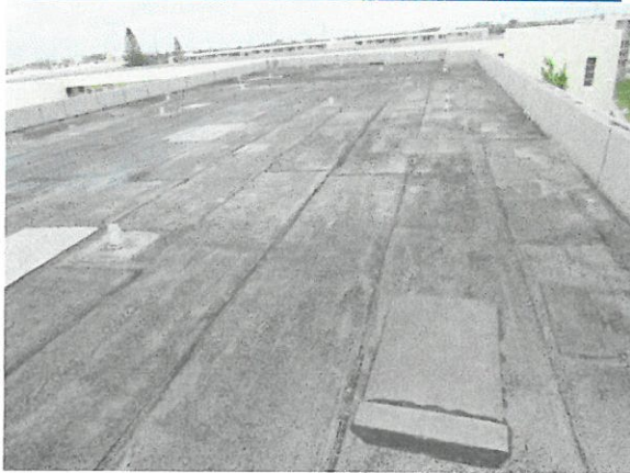
Reinforced Concrete Roof Deck
