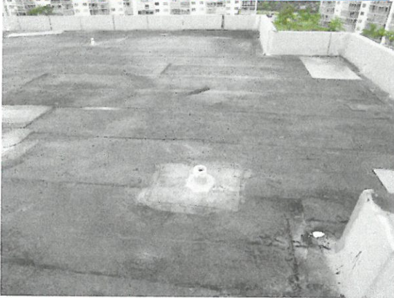
Reinforced Concrete Roof Deck
