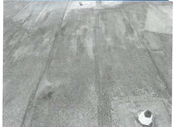
Reinforced Concrete Roof Deck
