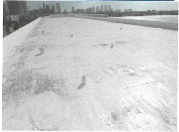
Reinforced Concrete Roof Deck
