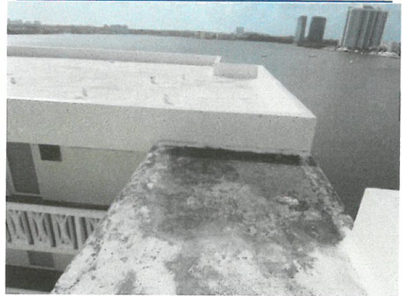
Reinforced Concrete Roof Deck
