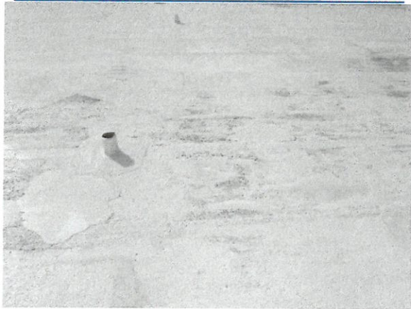
Reinforced Concrete Roof Deck
